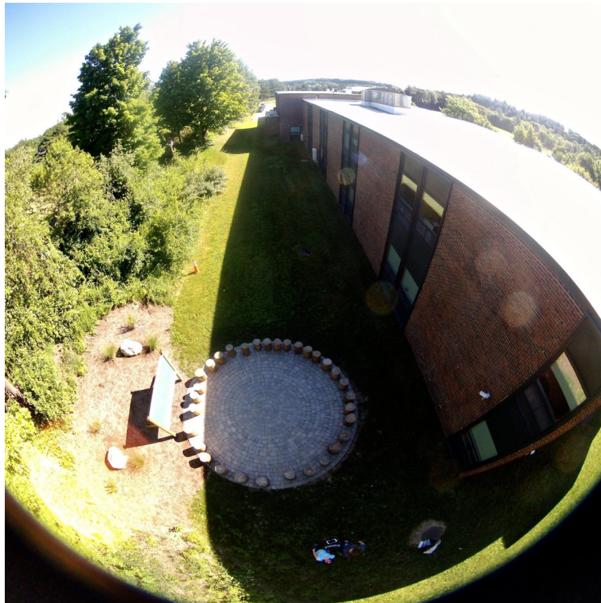
The outdoor classroom was completed during the last year through the support of multiple community members. (Courtesy Photo)
