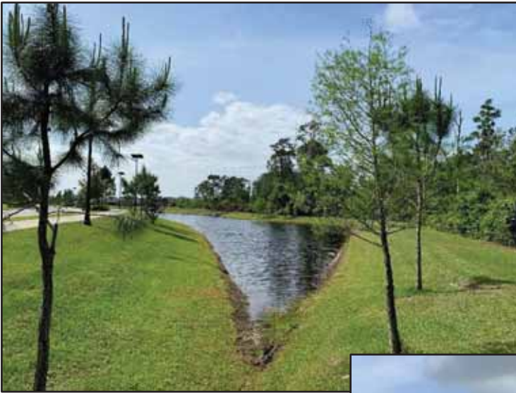
Pond scum remains in Pond 42
