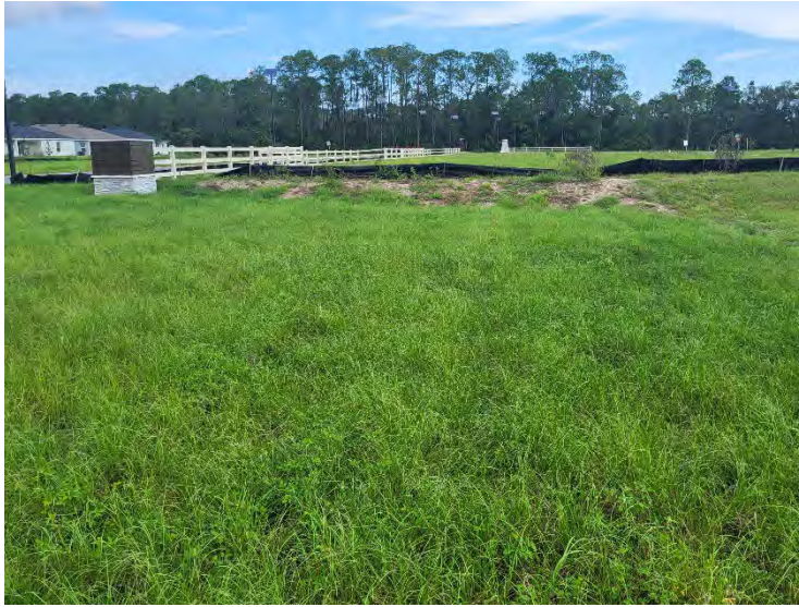
Location 4: Berm lacking turf.
