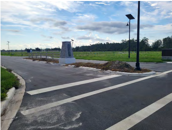
Location 13: Center Island not completed.
