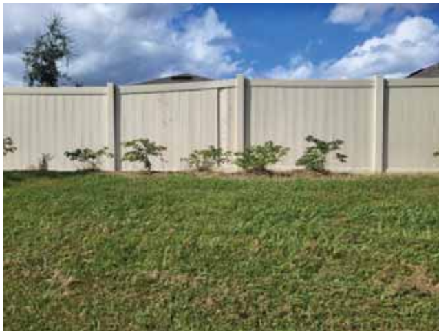
Location 2 – Repair existing fence and replace missing or damaged panels. Re-plumb fence
