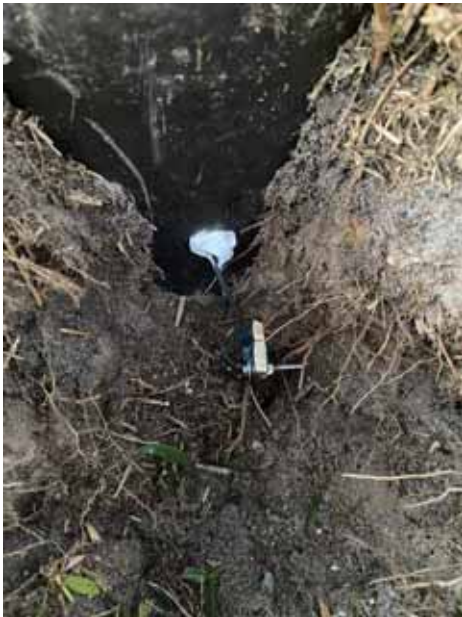
GND wire comes out 5" below the surface
