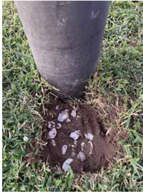
Hole filled with rocks and soil mix and compacted.
