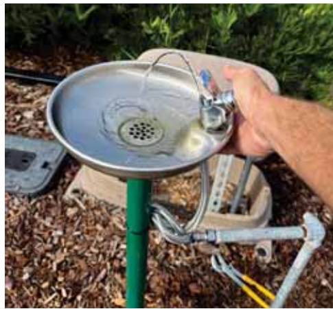
Goldcrest Loop Playground fountain repaired
