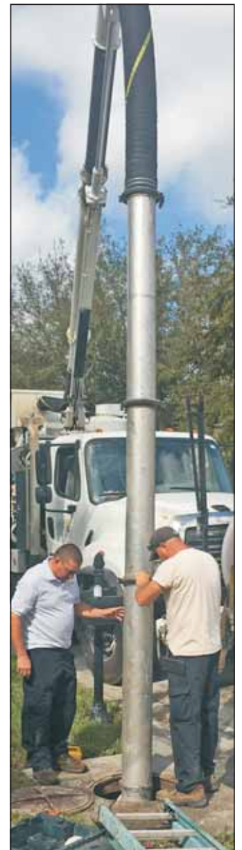
Top photo shows pump at left powering hoses to move water from pond to wetlands in background. At right, vacuum removes water, sand and muck from base of street stormwater drain in front of homes. Photo below shows wheeled camera that rolls through pipes and shows activity, such as water turbulence below bottom.
