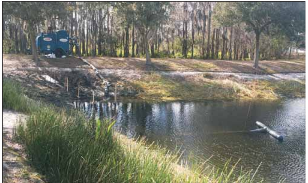
Top photo shows pump at left powering hoses to move water from pond to wetlands in background. At right, vacuum removes water, sand and muck from base of street stormwater drain in front of homes. Photo below shows wheeled camera that rolls through pipes and shows activity, such as water turbulence below bottom.
