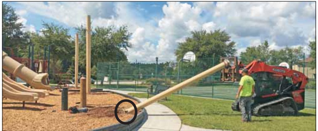
The poles that held up the cover above the children's play area in Ballantrae Park were recently removed. Note inside of circle the thin flange at base of pole that held it in place at ground level with six large screws.
