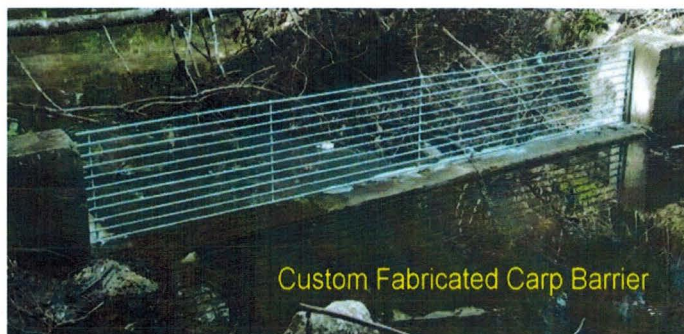
Picture 2. Carp Containment Barrier on Pond Outfall
