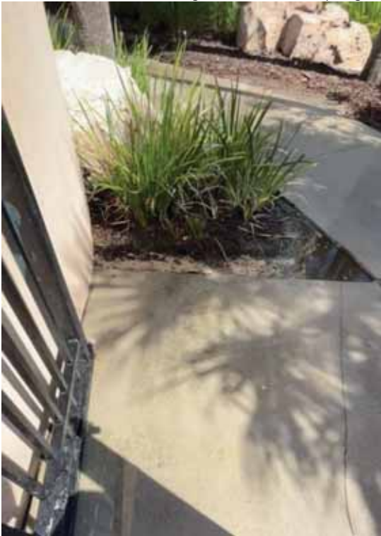
Slide entrance drainage and landscaping- Before
