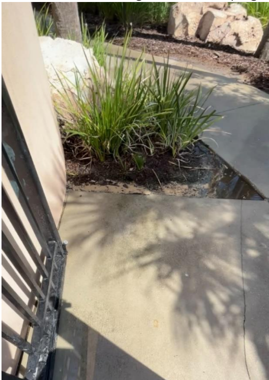
Slide entrance drainage and landscaping- Before
