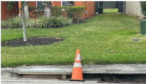
Inlet tops – 4 repaired
