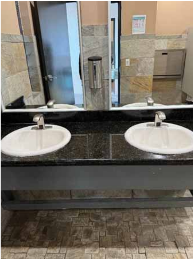
Replaced bathroom sink faucets
