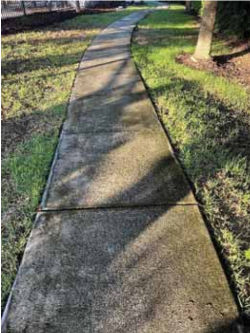
Playground Walkway before
