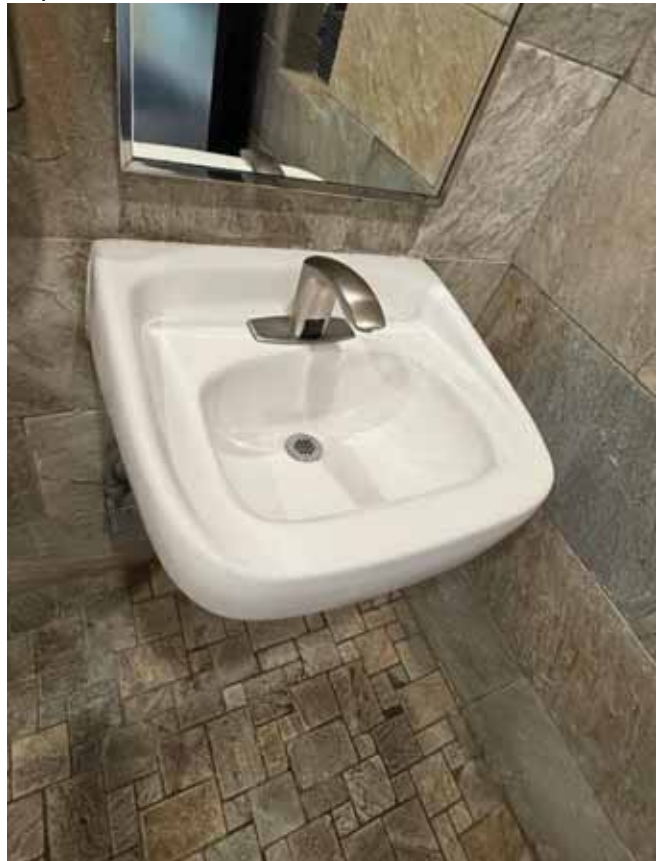
Replaced bathroom sink faucets
