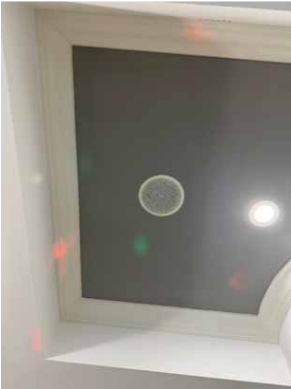
Clubhouse ceiling caulked
