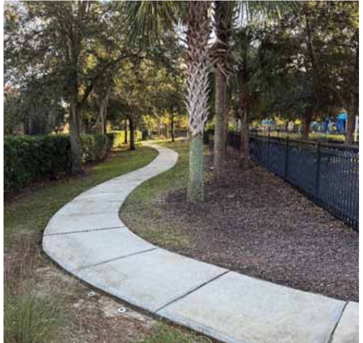
Playground Walkway after
