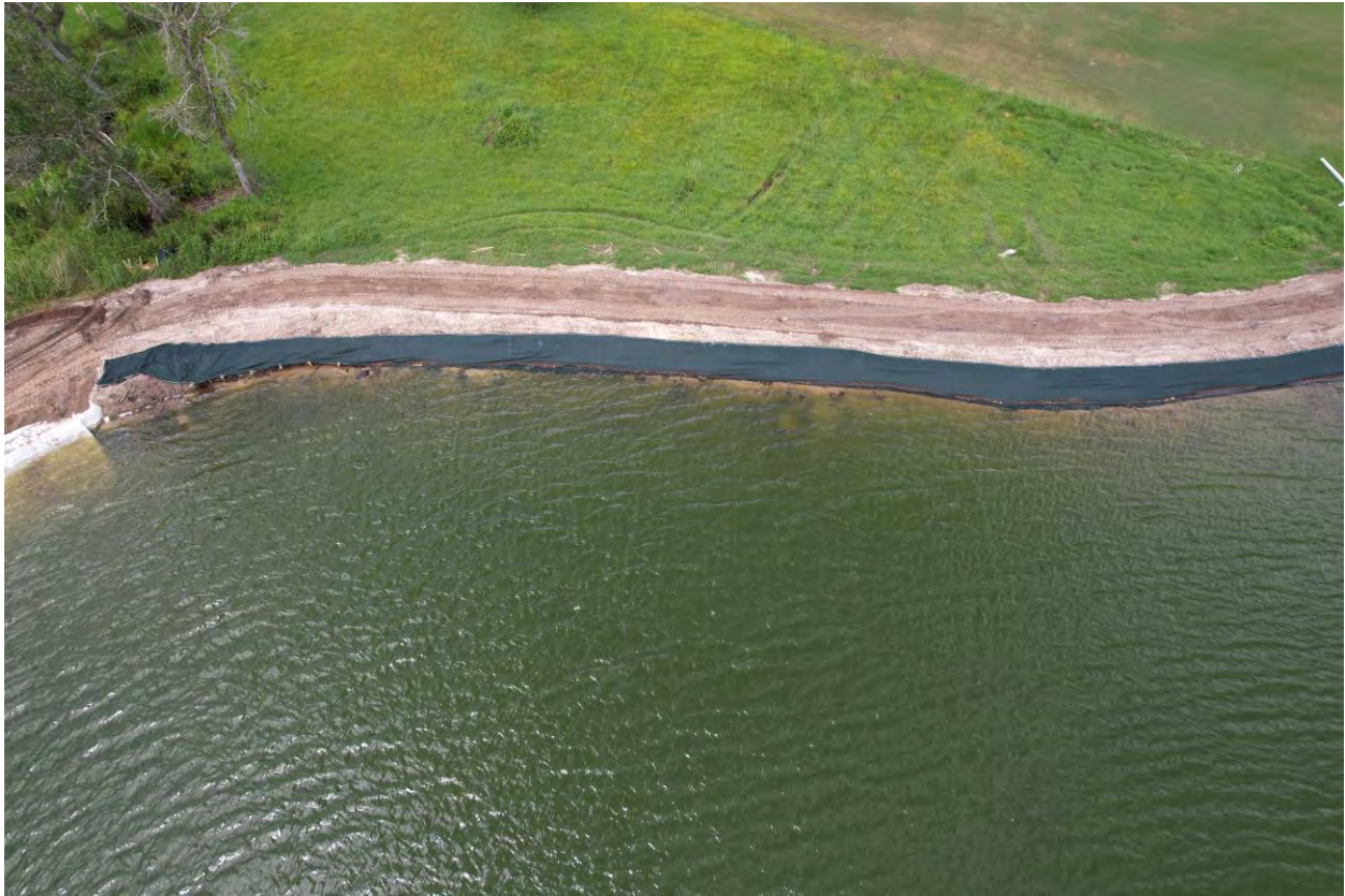
Fig 8 Dirt Coverage on GCL / Installing SOX
