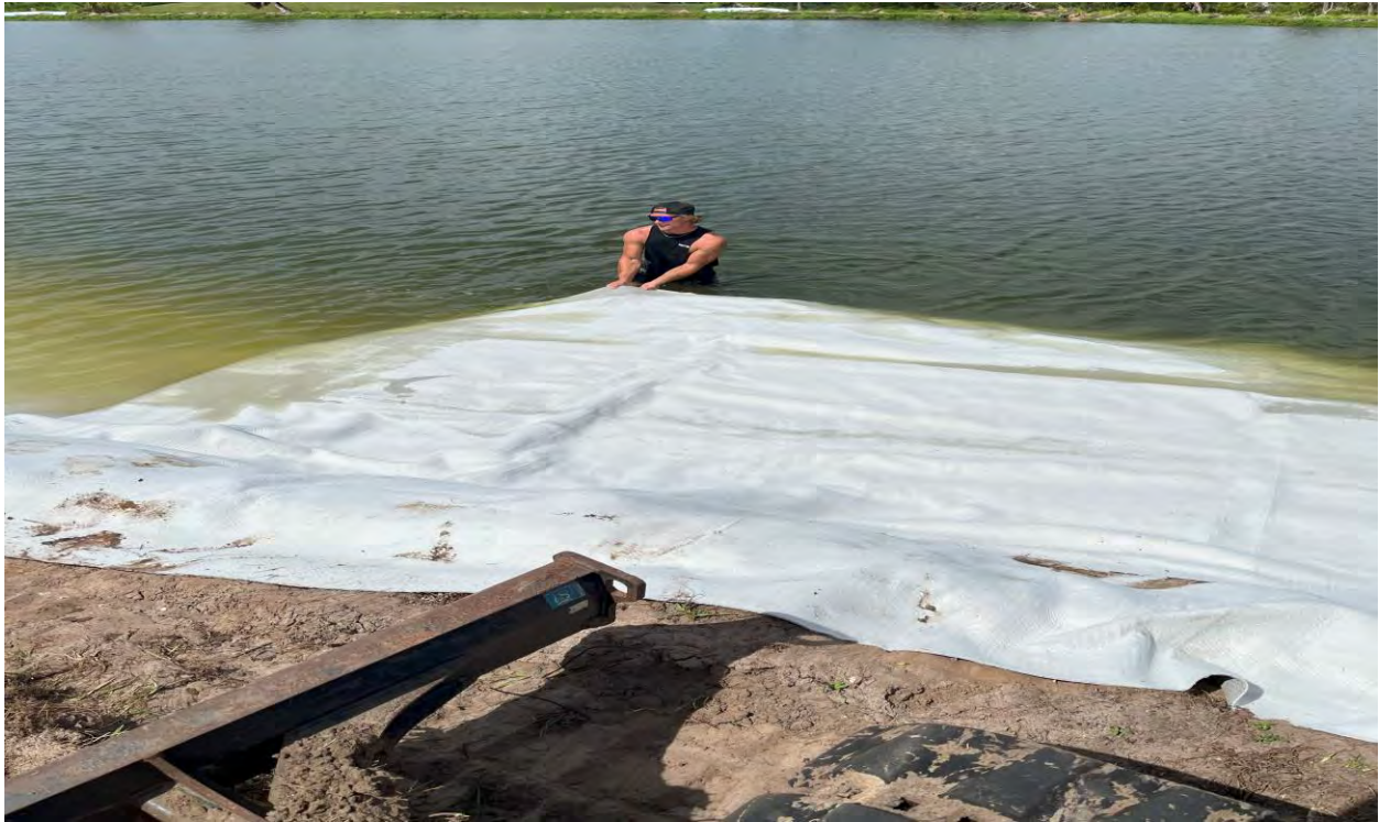
Fig 6 Installing GCL into water
