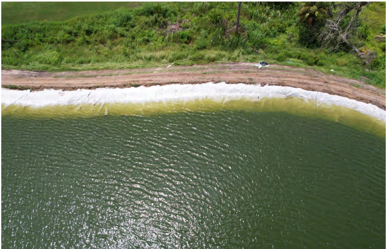
Fig 7 GCL Installed
