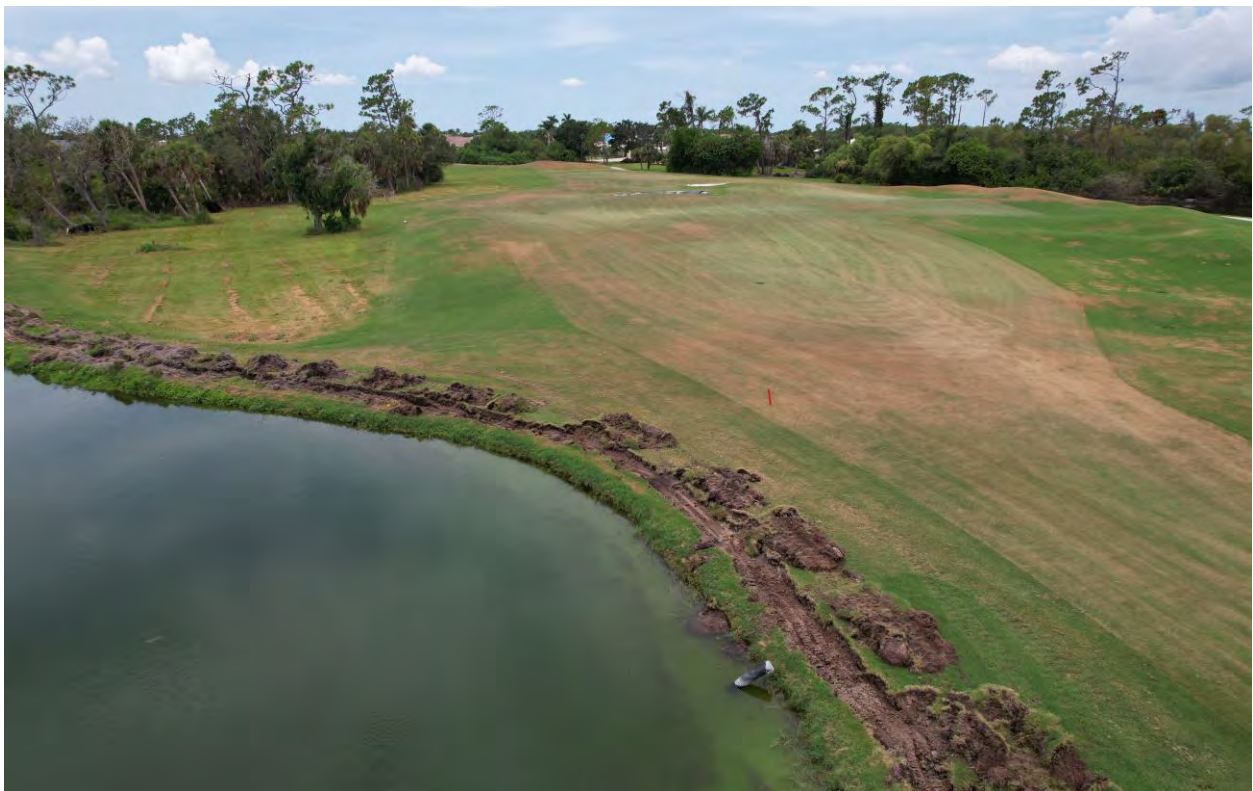
Fig 3 – Trench for GCL
