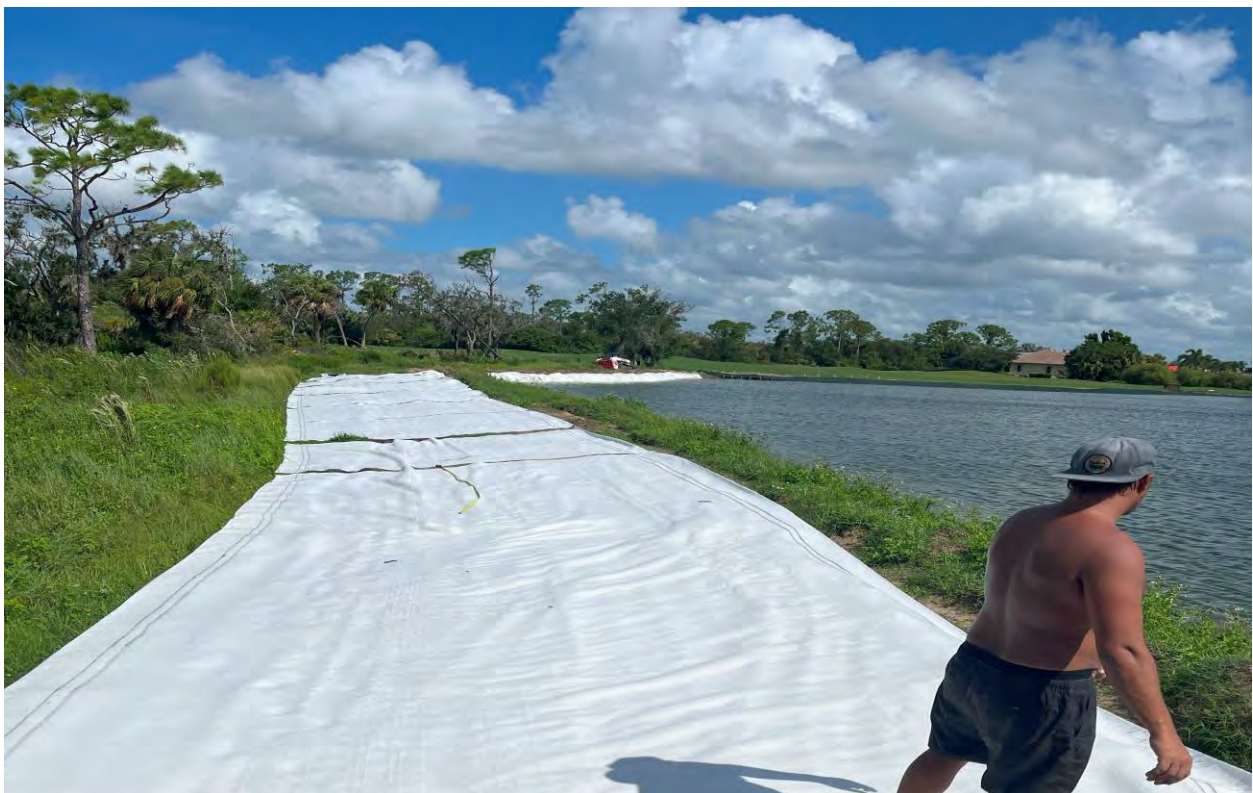
Fig 5 Cutting GCL to Length
