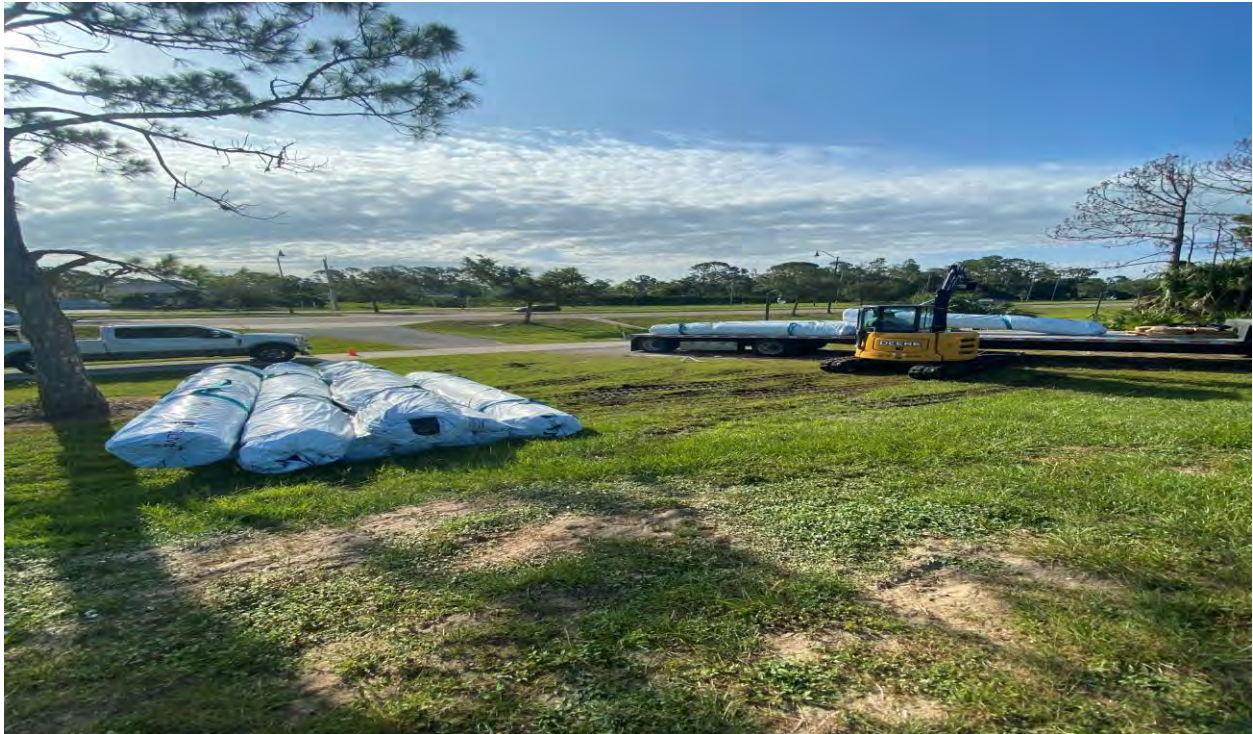
Fig 4 Unloading GCL
