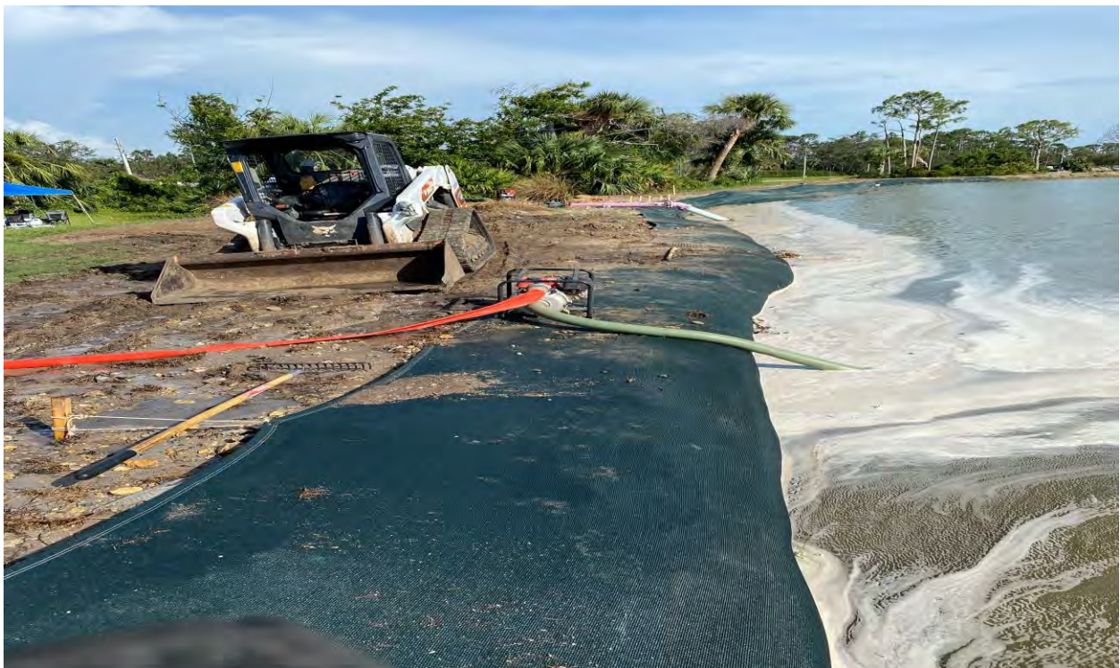
Fig 9 Pumping material into SOX
