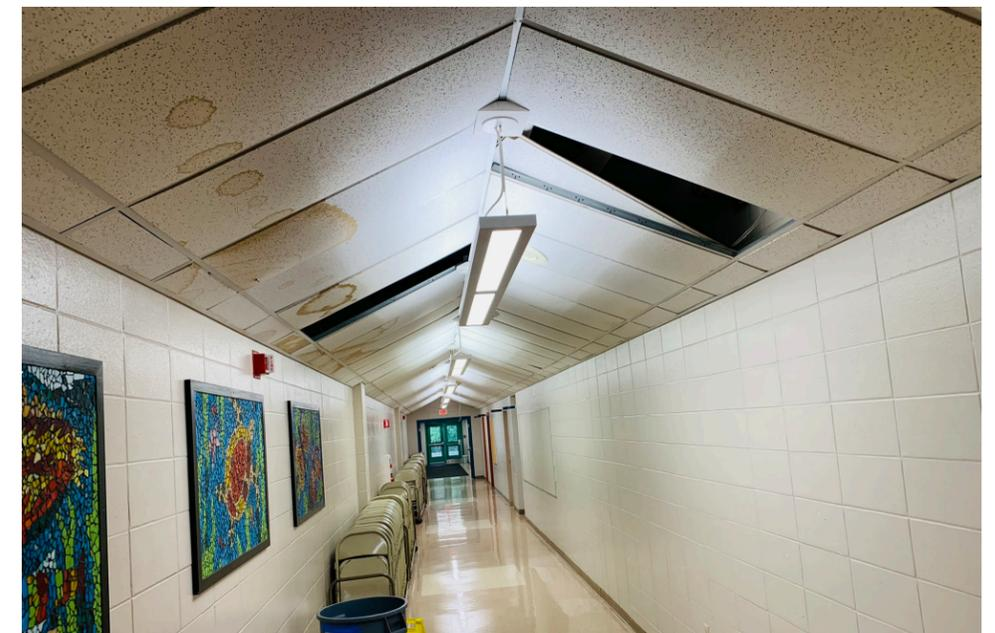
Water damaged ceiling tiles were noted in several locations throughout the school. This may be indicative of a leaking roof. Further assessment is required.
