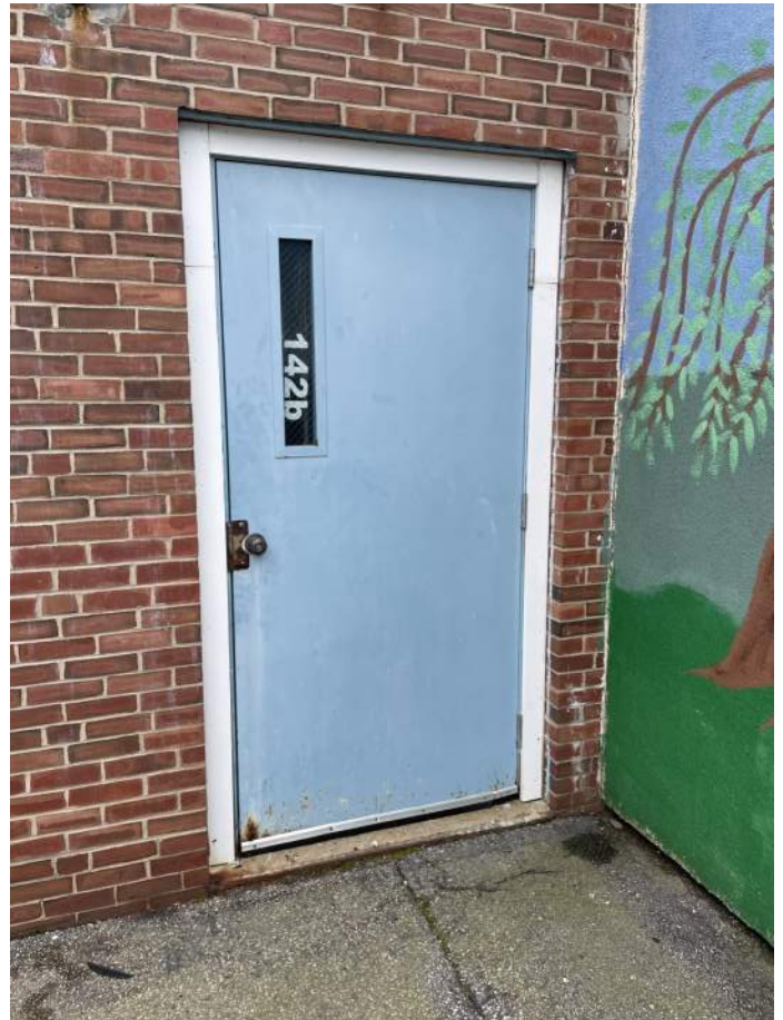
Exterior Door in Poor Condition.
