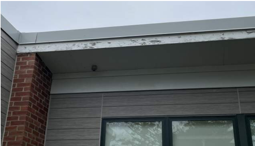
Roof Fascia Trim Requiring Repair.
