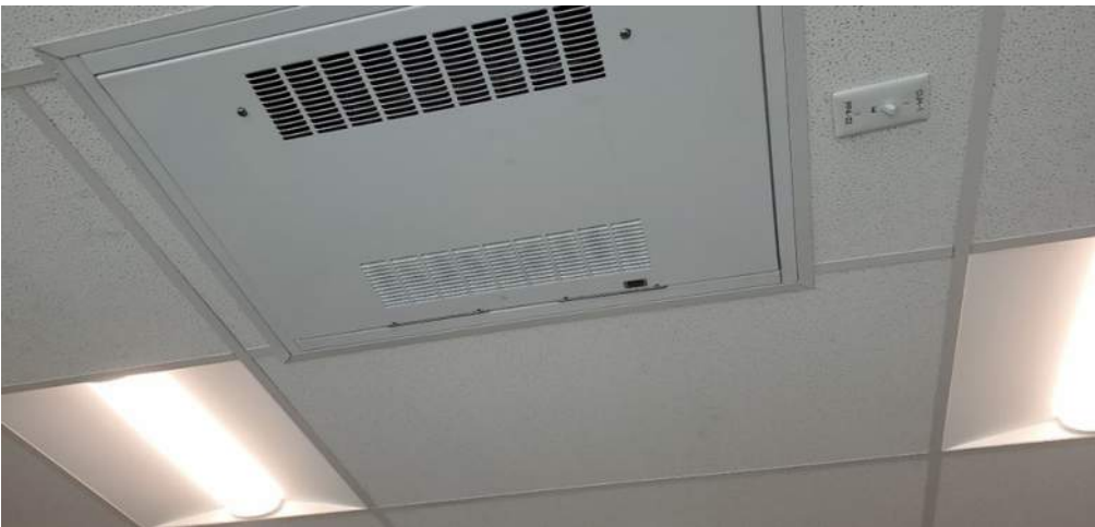
Cabinet Unit Heater in Vestibule.
