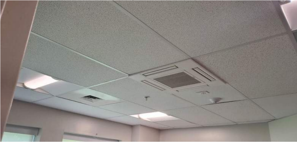
Fan coils in the Administrative Addition.
