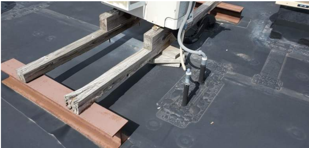
Failing Condenser Unit Supports.
