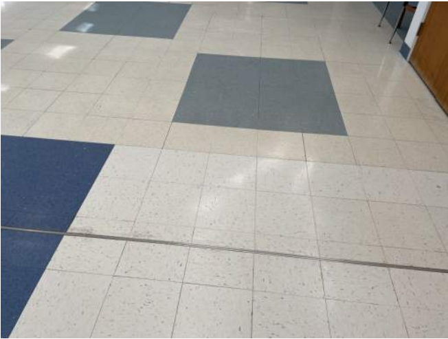
Vinyl Flooring on Poor Condition.
