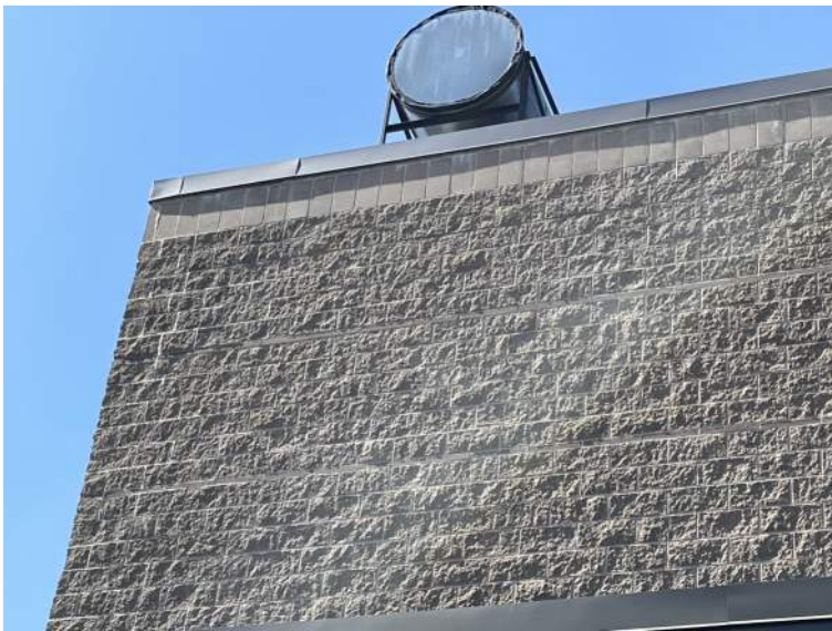
Efflorescence at Auditorium Roof Edge.
