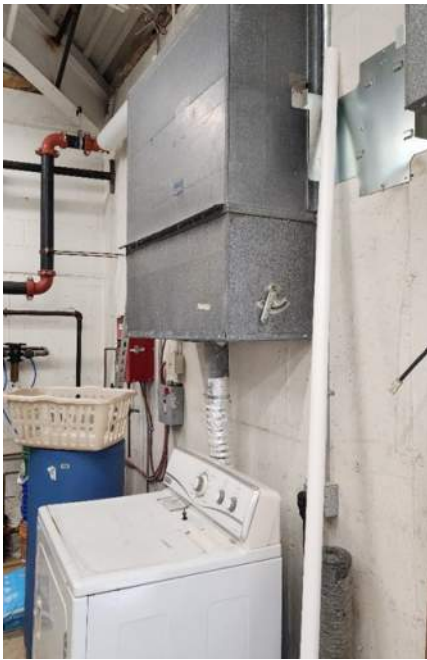
Non-Compliant Dryer Vent.
