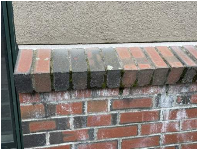
Efflorescence and Mildew at Brick Veneer.
