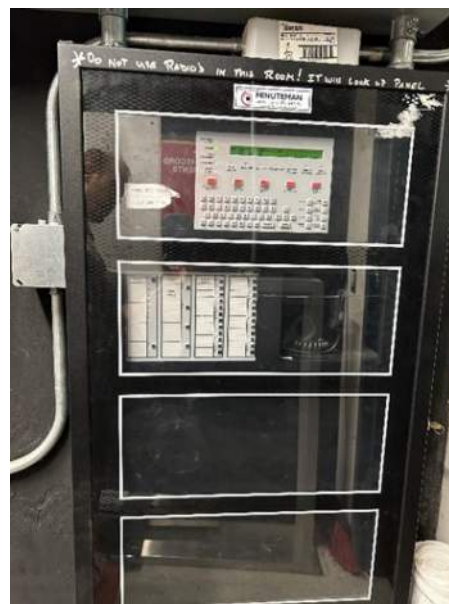
Fire Alarm Control Panel.
