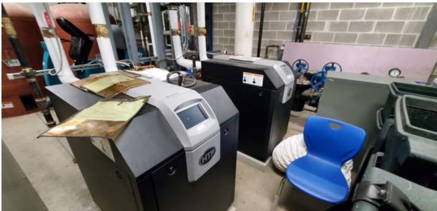
Instantaneous Domestic Hot Water Heaters.
