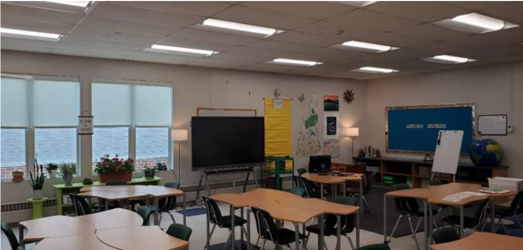
Typical Classroom with Fin Tube Radiation and No Cooling.
