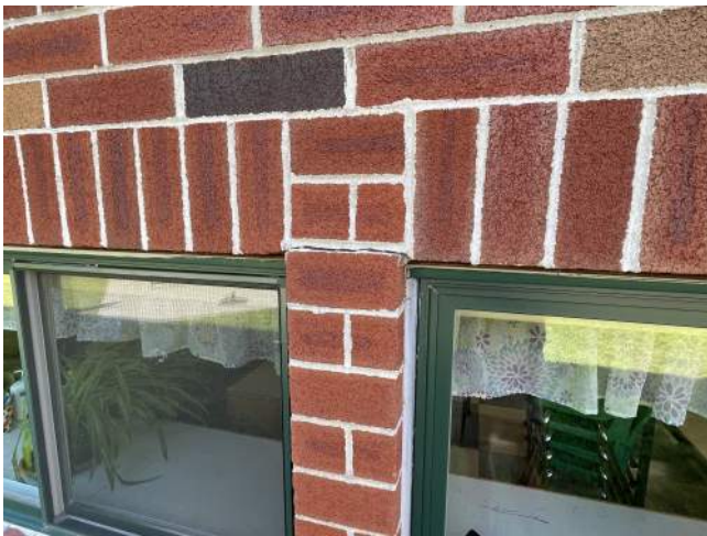
Cracking of Brick Veneer at Window Head Conditions.
