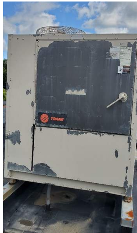
ACCU in Poor Condition.
