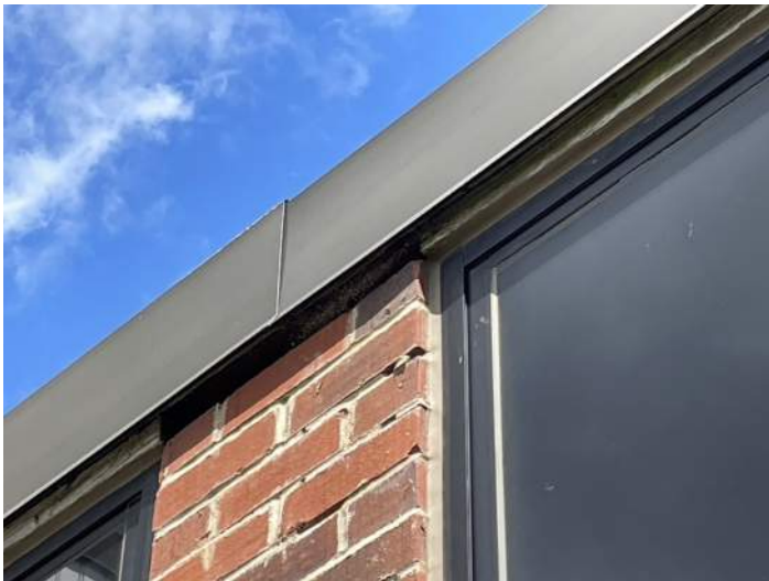
Wood Blocking in Poor Condition.
