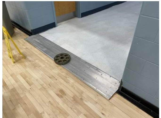
Gym Transition Strip in Poor Condition.
