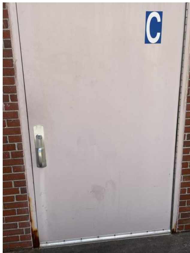
Exterior Door Corrosion.
