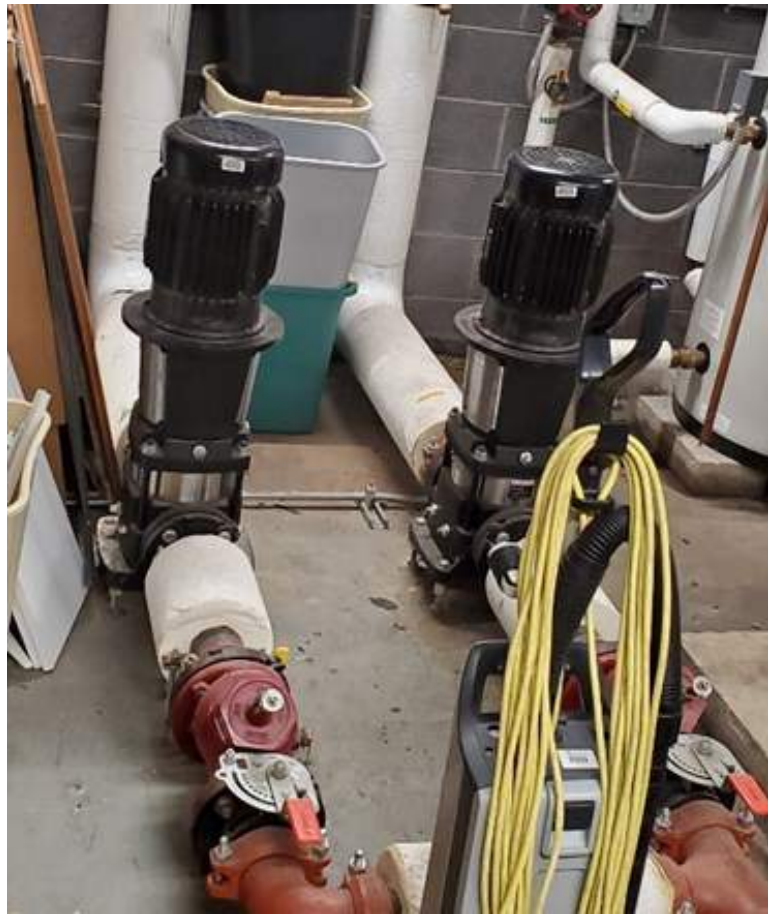
Secondary Loop Boiler Pumps.
