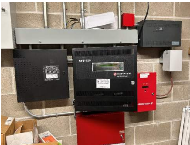
Fire Alarm Control Panel.
