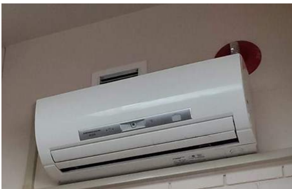
Existing Wall Mounted Fan Coils.
