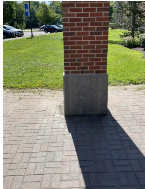
Main Entry Area Susceptible to Ponding.
