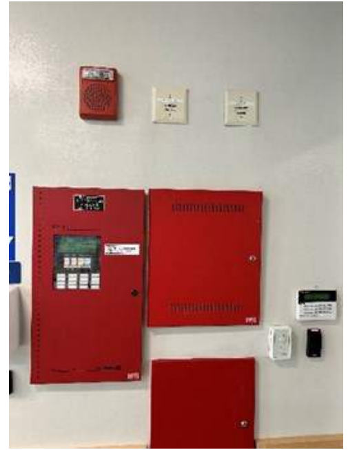
Main Fire Alarm Control Panel.
