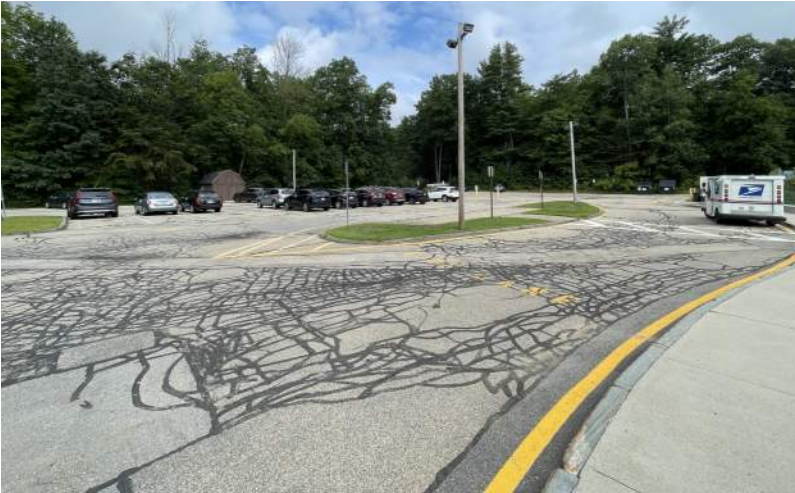
Asphalt Paving in Poor Condition.
