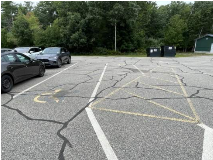
Asphalt Paving in Poor Condition.
