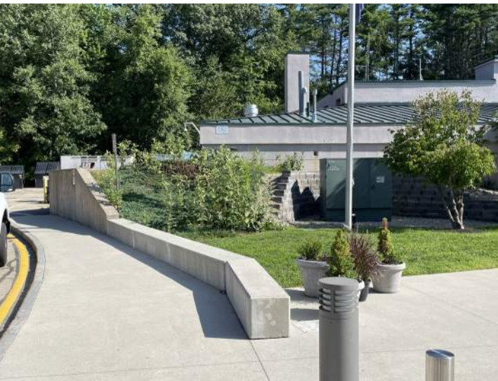
Berm Provides Easy Access to Roof, Gas Service, and Top of Transformer.
