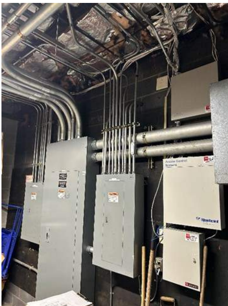
Electrical Main Distribution Panel.
