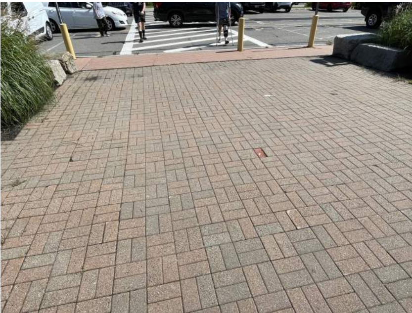
Main Entry Area Susceptible to Ponding.
