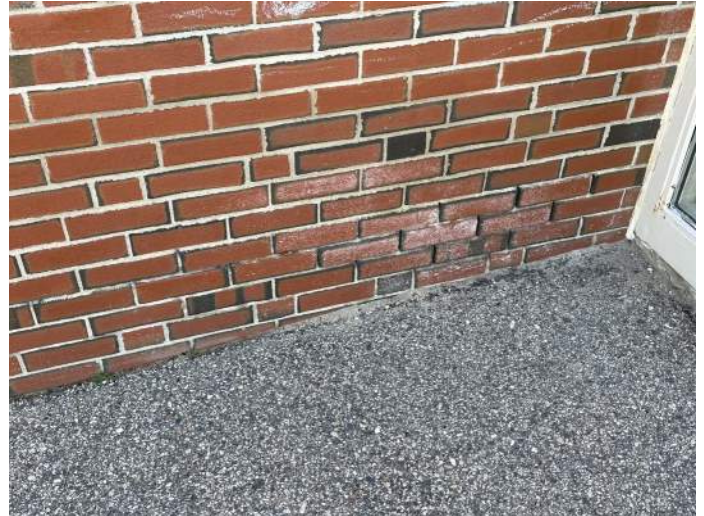
Brick Requiring Repointing.
