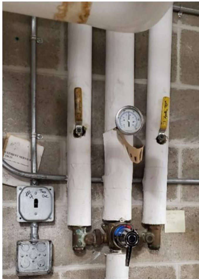
Thermostatic Mixing Valve.
