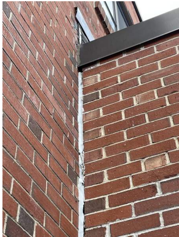
Sealants in Poor Condition.
