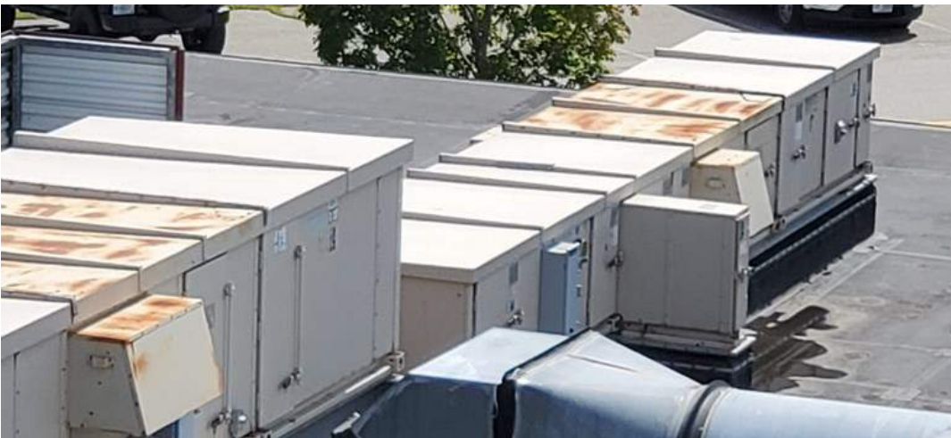
Condensate Pooling Adjacent to AHU-2.
