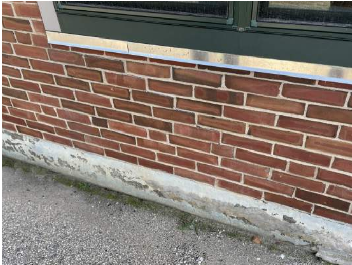
Concrete Foundation in Poor Condition.
