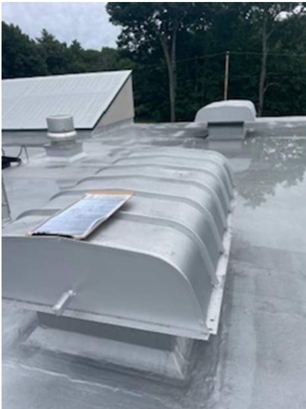
Gravity Ventilators.
