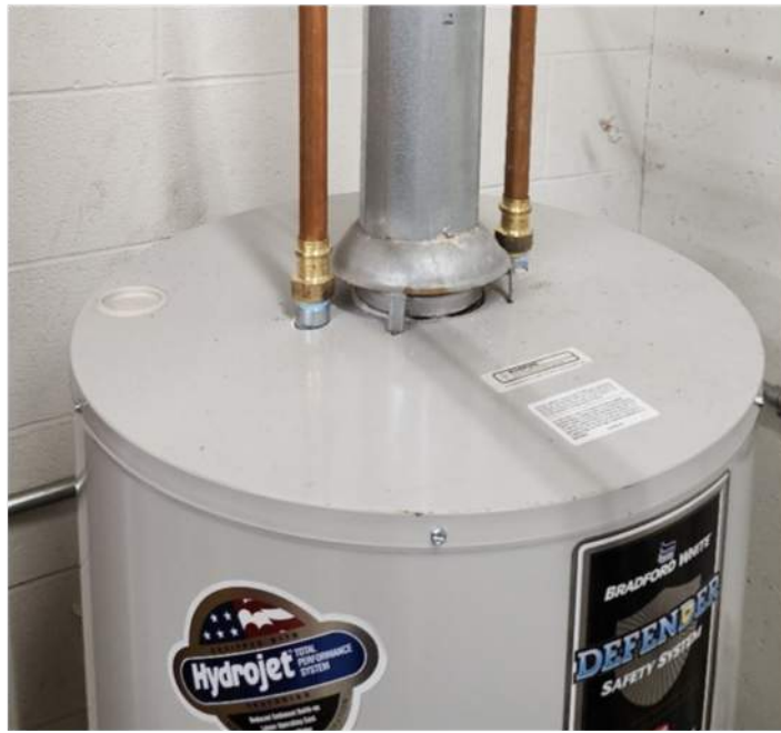
Domestic Hot Water Heater Vent.
