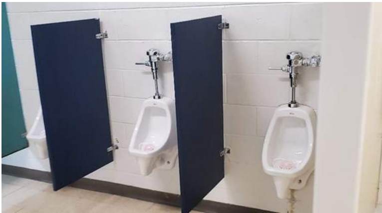
Manually Operated Fixtures in the Older Wings.
