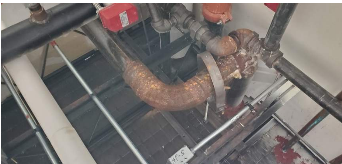
Corroded Fire Protection Piping in Compressor Room.
