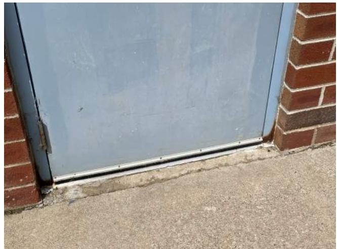
Corrosion at Exterior Doors.
