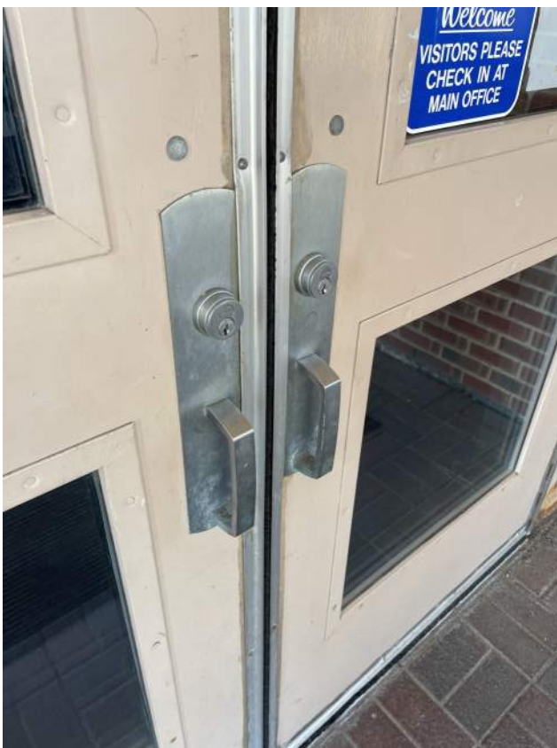
Exterior Door Hardware Recommended to be Replaced.
