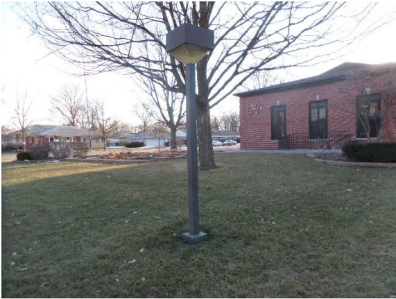
Typical pole-mounted exterior light fixture with yellowed lens, scheduled for replacement.
