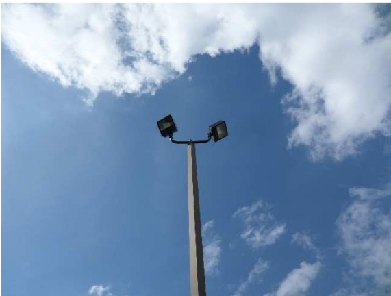
Typical pole-mounted exterior light fixture with yellowed lenses and showing signs of rust, scheduled for replacement.
