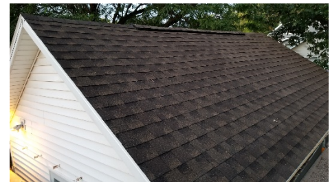
The garage before, during and after a new roof was installed by Kimberly High School students.
