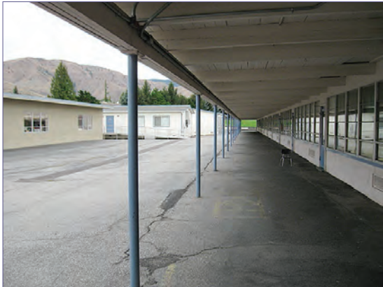
Portables on left house overflow students. Every class had a door to outside, which is a security concern. Single pane windows line the exteriors. The single corridor design 120-yards long causes traffic-flow problems for students and staff between class.
