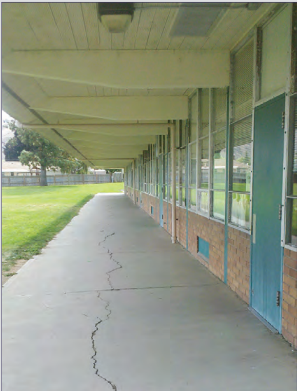
Lincoln’s exterior walls lack insulation, windows are single pane and lack energy efficiency. Exterior doors to every classroom is a security concern.
