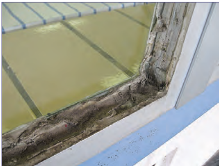
A deteriorated window frame.
