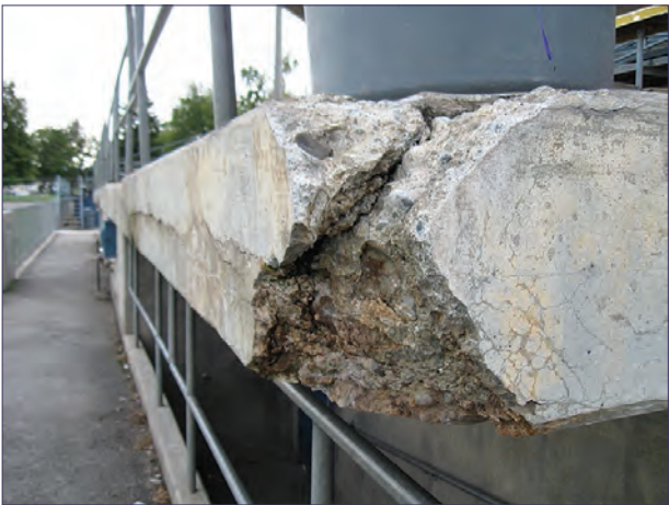
Concrete slab on outdoor bleachers also serves as roof to locker rooms. The slab is deteriorating.
