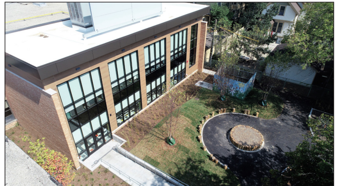
Aerial image of the Holmes expansion, courtesy of Bulley & Andrews.
