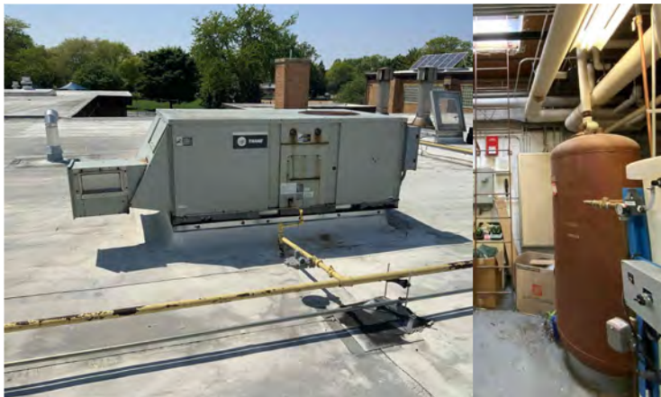
Rooftop Unit and Boiler | Lifespan 20-40 years
