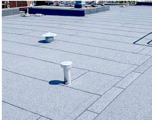
Typical Modified Bitumen Roof | Lifespan 15-20 years
