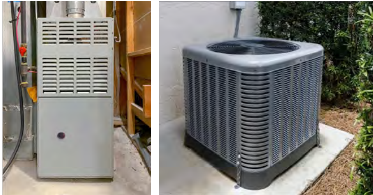
Furnace and Condensing Unit | Lifespan 15-25 years
