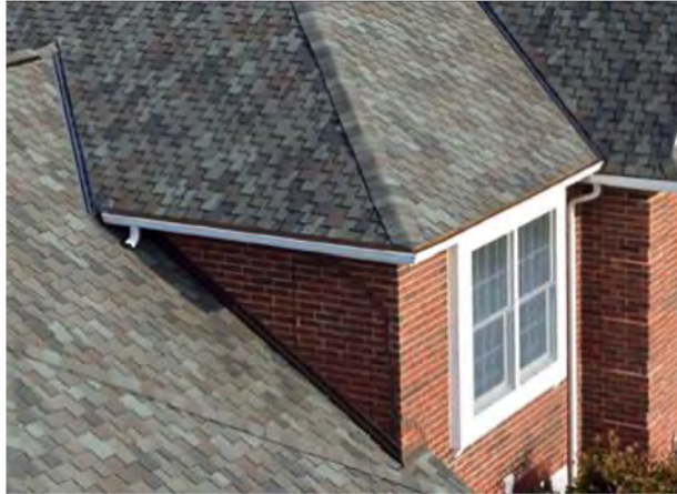
Typical Shingle Roof | Lifespan 15-30 years
